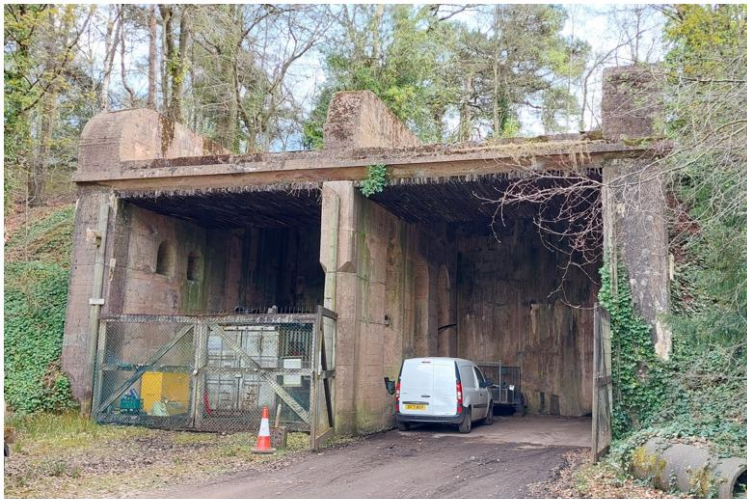
The proofing range butts, into which guns were fired.
